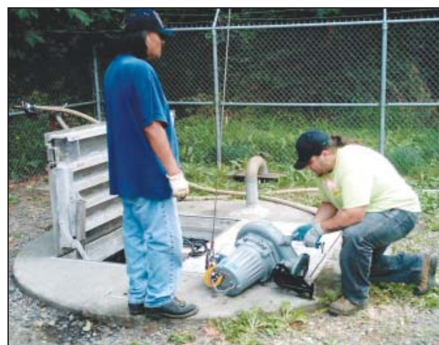
The Utility District's Dewey Miller and Riley Patterson service a sewer pump at Lift Station #1.
